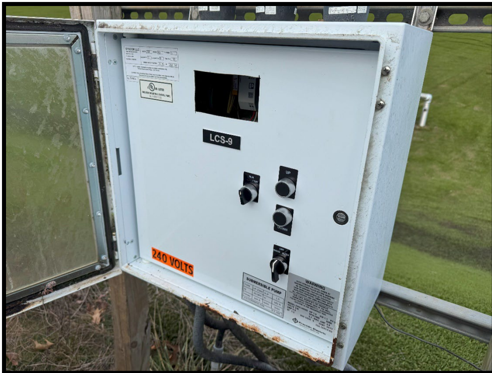
Photograph 2: View of missing display in LCS-9 panel.
