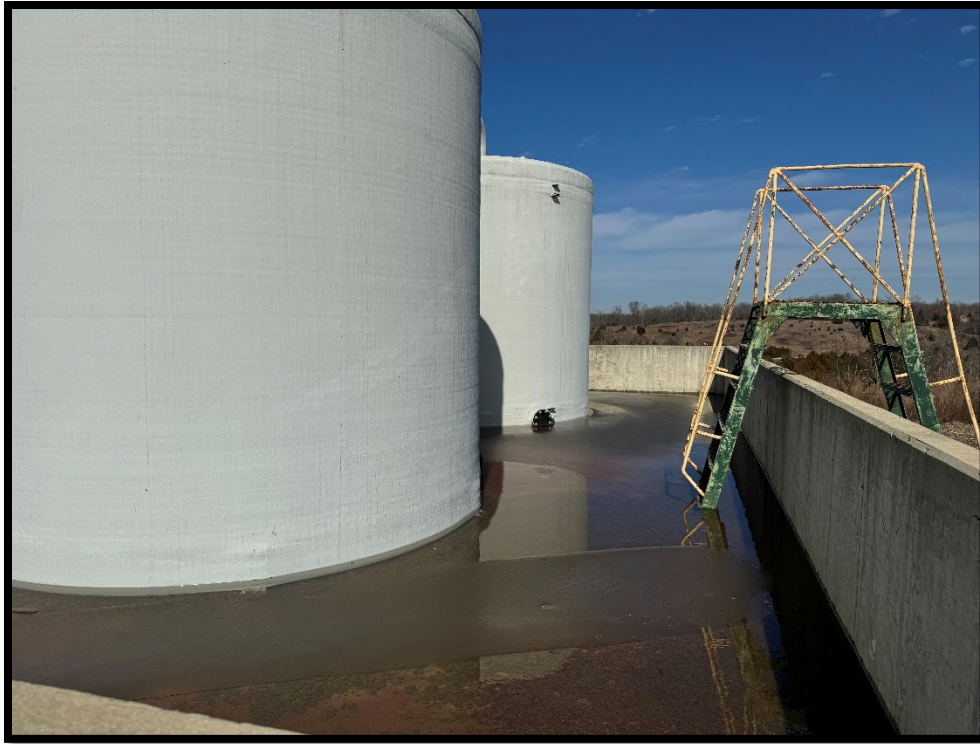
Photograph 1: View of approximately 7.5 inches of stormwater in secondary containment.
